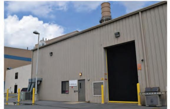
After a near-miss incident involving a steel rolling door free-falling, the plant decided to replace the existing rolling steel doors with the PerforMax MaxSpeed rubber door. With its built-in safety brake, the chance of door free-fall is completely eliminated. In addition, there is no downtime due to accidental impacts with the breakaway design of the doors.
